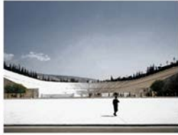
Panathenaic Stadium, Athens, Greece, 1959
